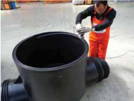
Ring on the inspection chamber shall be cut off primarily.
