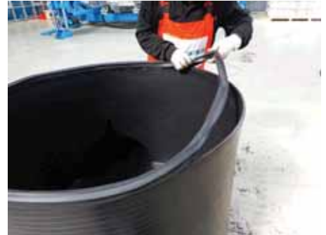
Upon spreading liquid soap in conical top piece seal groove and seal surface, two pieces are joined.
